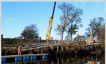
Piles were installed along the river's edge to serve as support for the two linkspan bridges and also so that the pontoons could be attached to them. Between the two sites, a total of eight piles each measuring 457mm x 13m were installed. Reinforced concrete foundations were also constructed by TMS at both sites using our multi-disciplinary marine civil engineering resources.
