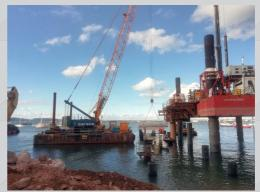
A significant challenge experienced during the project was the variable and unpredictable nature of the local geology, which made piling considerably complex. However, once the piles were installed, pre-cast concrete units were added before an in-situ reinforced concrete deck was poured. Once completed, the original rock armour was replaced.
